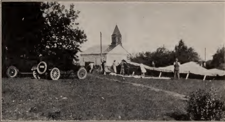
SETTING UP THE CONFERENCE TENT AT THE MISSION HOUSE, WISCONSIN
